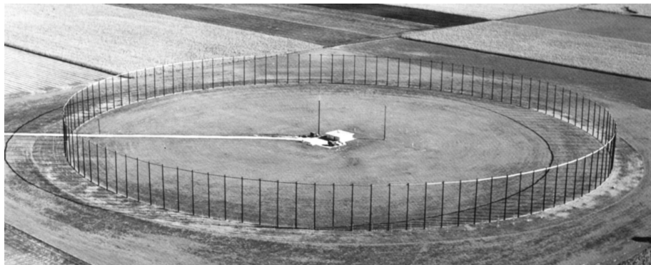
FIGURE 1 Wullenweber Antenna Array in existence at the Bondville Road Field Station of the University of Illinois at Urbana-Champaign from 1955 to 1980.
